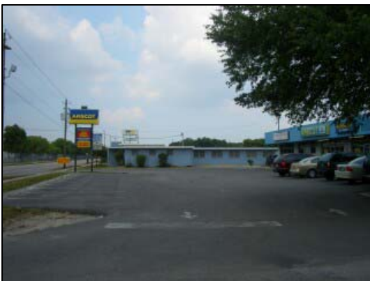
Parking Lot From E.
